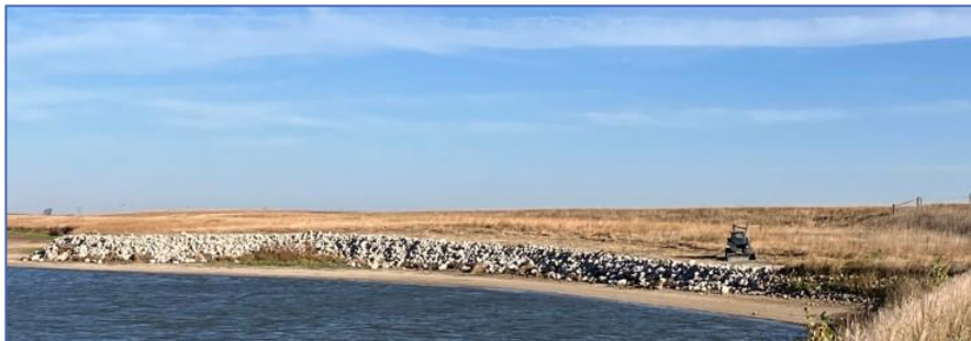
MARC dam being upgraded with Class B riprap.
